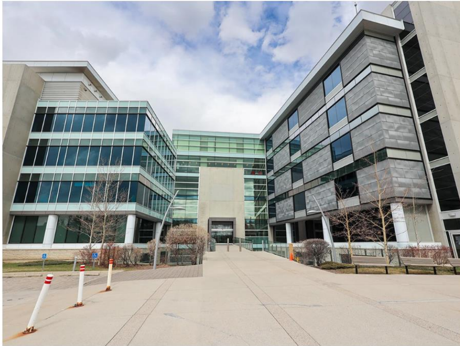
The former SMART Technologies building near the University of Calgary will become a Charter Hub, housing a number of charter schools. Gavin Young/Postmedia
